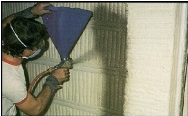
Fiber wall being sprayed with ITC-100 HT
