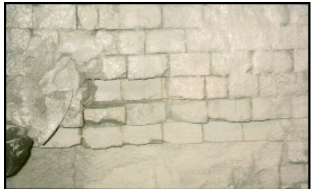
Brick wall being repaired with ITC-200 EZ over ITC-100
